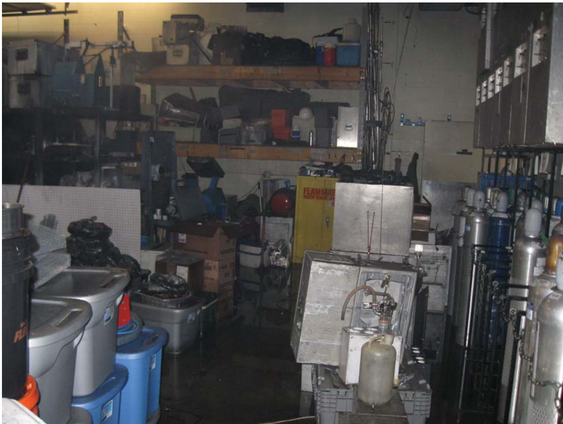
Figure 3 – Rear of the shop area, no fire extension to other items in the shop.
