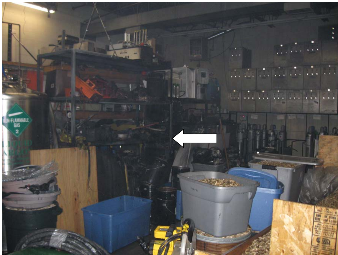
Figure 1 – Fire was located on the other side of this racking.
